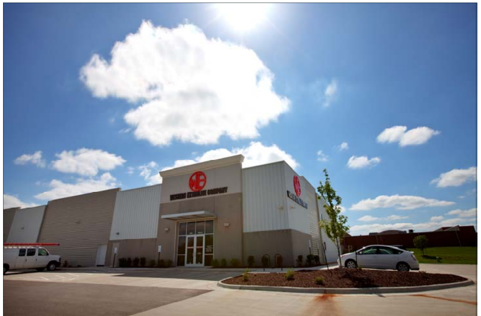
The Daikin system installed in Western Extralite’s Lawrence facility was named the city’s first LEED certified private business, and was awarded LEED Silver certification in January 2010. Owners cite the energy consumption of the 20,000-square-foot space is similar to the energy used in their old 12,000-square-foot building.
